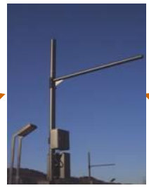
Utility Pole for Base Station
